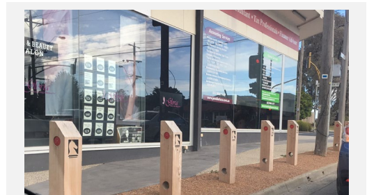
Timber Bollard: Access restriction, unknown containment, impact behaviour unknown- deemed frangible in one direction.
